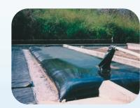
Under proper conditions, Geotube<sup>®</sup> MT units can also be used in drying beds to increase capacity.
