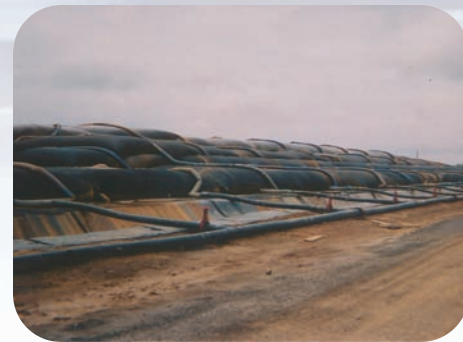
Lagoon cleanup can be a problem and a liability. Geotube® technology simplifies the dewatering process.
