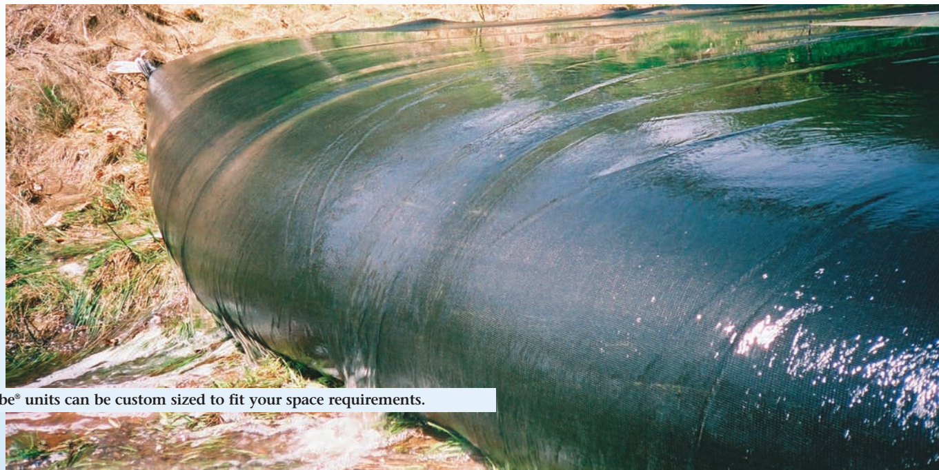
Lagoon cleanup can be a problem and a liability. Geotube® technology simplifies the dewatering process.
